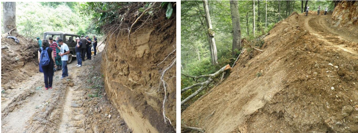
Vertical cuts and loose, sidecast fills used in local Adjara new road construction are both likely to cause some instability problems over time.
