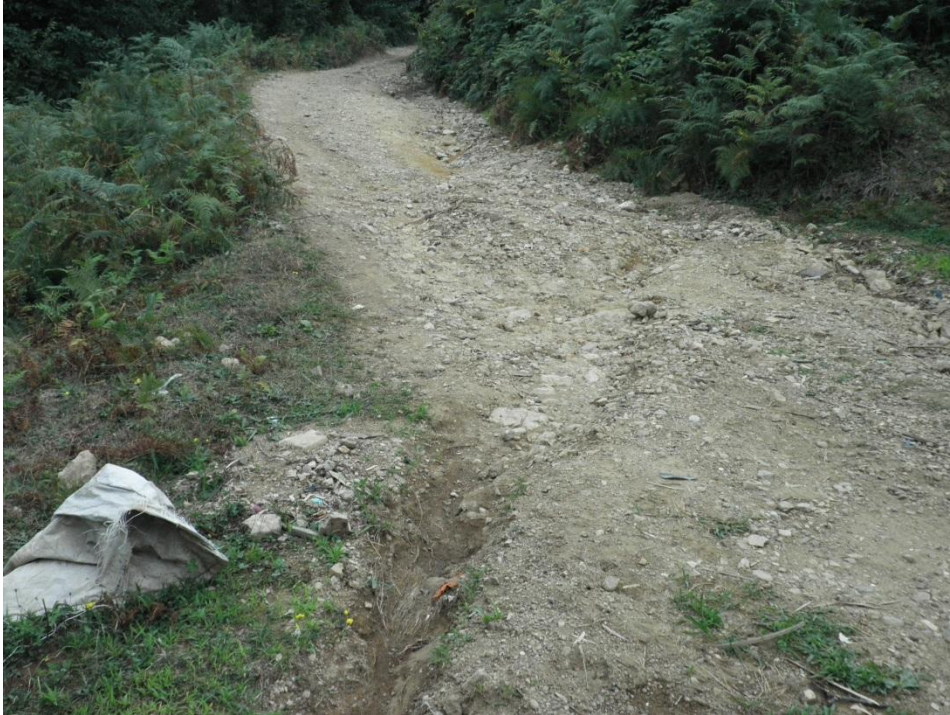
Photo of a road surface drainage dip that is working but that needs to be deepened to function during a major storm
